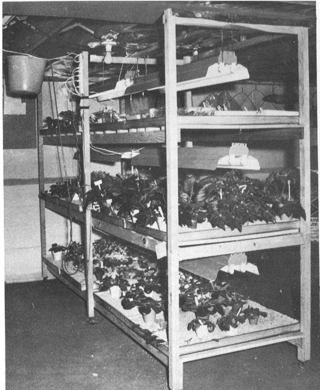
Shelves and lamps for experiment in phytoillumination
