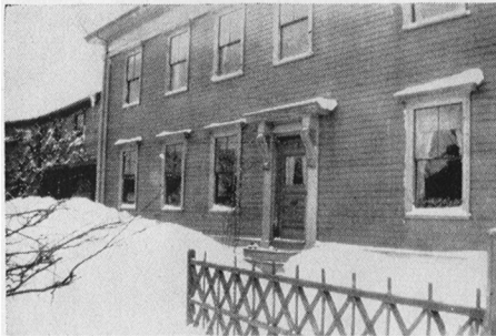
Sheltered Porch in Distance
